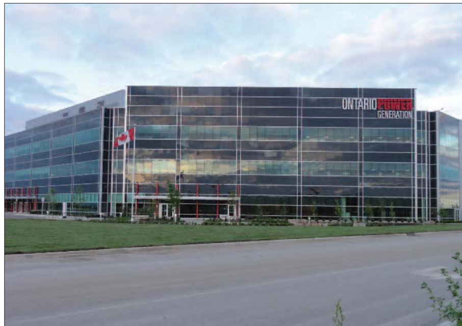
The Darlington Energy Complex
